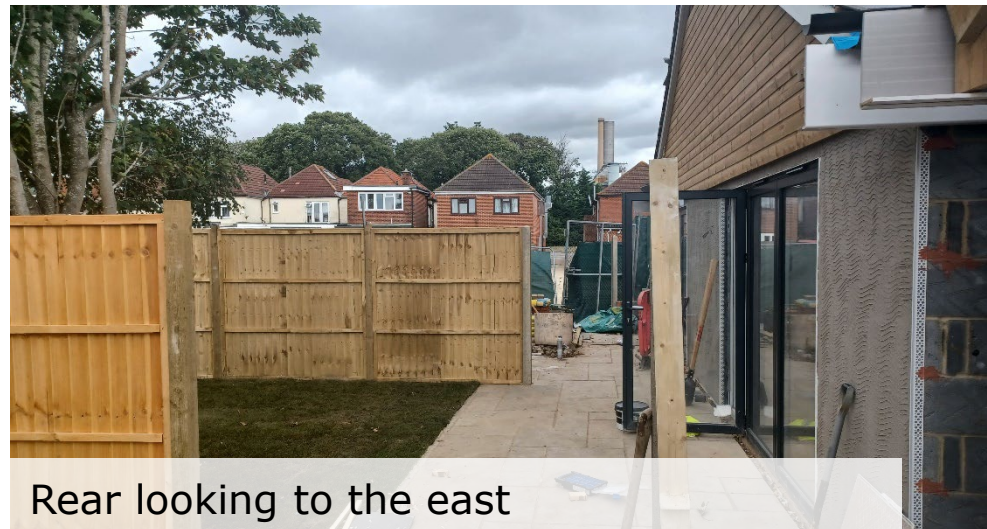
Eastern end of site
