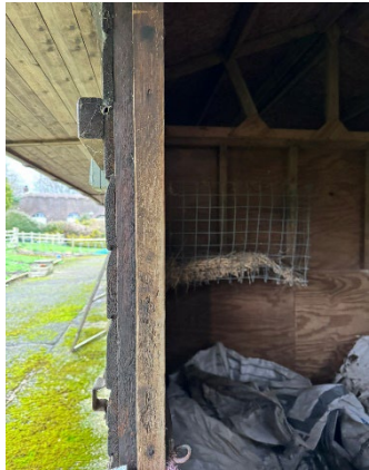
Construction of existing stable
